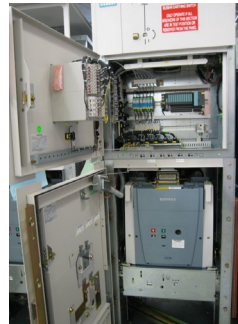
Converters mounted inside Switchgear
