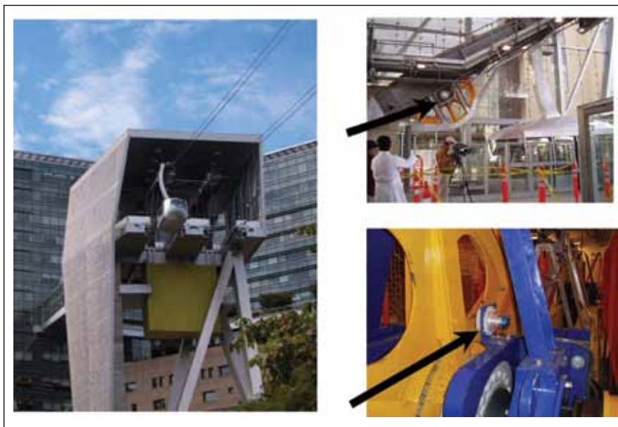
Figure 10—Portland aerial tram uses fiber optic rotary encoders.
